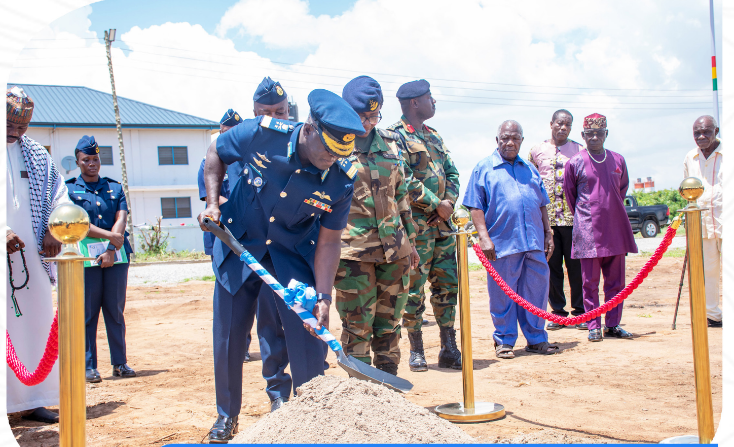
THE CHIEF OF THE AIR STAFF, AVM FAK BEKOE CUTTING SOD FOR THE CONSTRUCTION OF A THREE STOREY, 24 STUDIO APARTMENTS FOR AIRMEN AT AIR FORCE BASE ACCRA.
